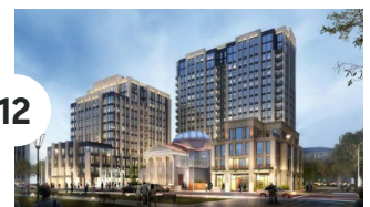
12 PARK VIEW TOWERS 252 N FIRST STREET SAN JOSE
